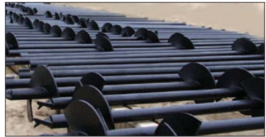
Line-UP: 440 Winslow Geo Anchors await installation of the third phase of the Willow Park Marina development, Bethel Island, CA. When completed 1,100 anchors will provide the foundation for over 60 condominium units built in an area with a high water table.
